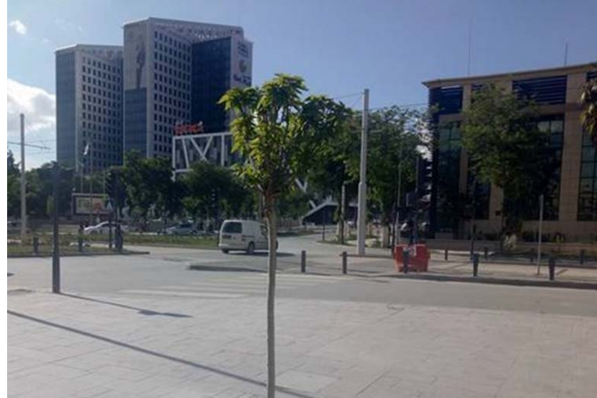
Photo (01): The “Al-Ali” commercial center
