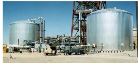
Tank direct storage of the "Solar Two" plant near Barstow, USA
